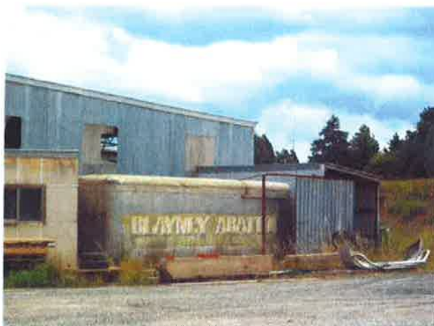
Old refrigerated van unit
